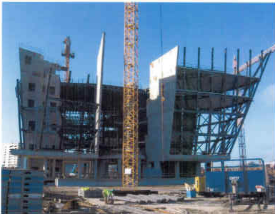
Photo 18 North Elevation (As at 30.09.10)
