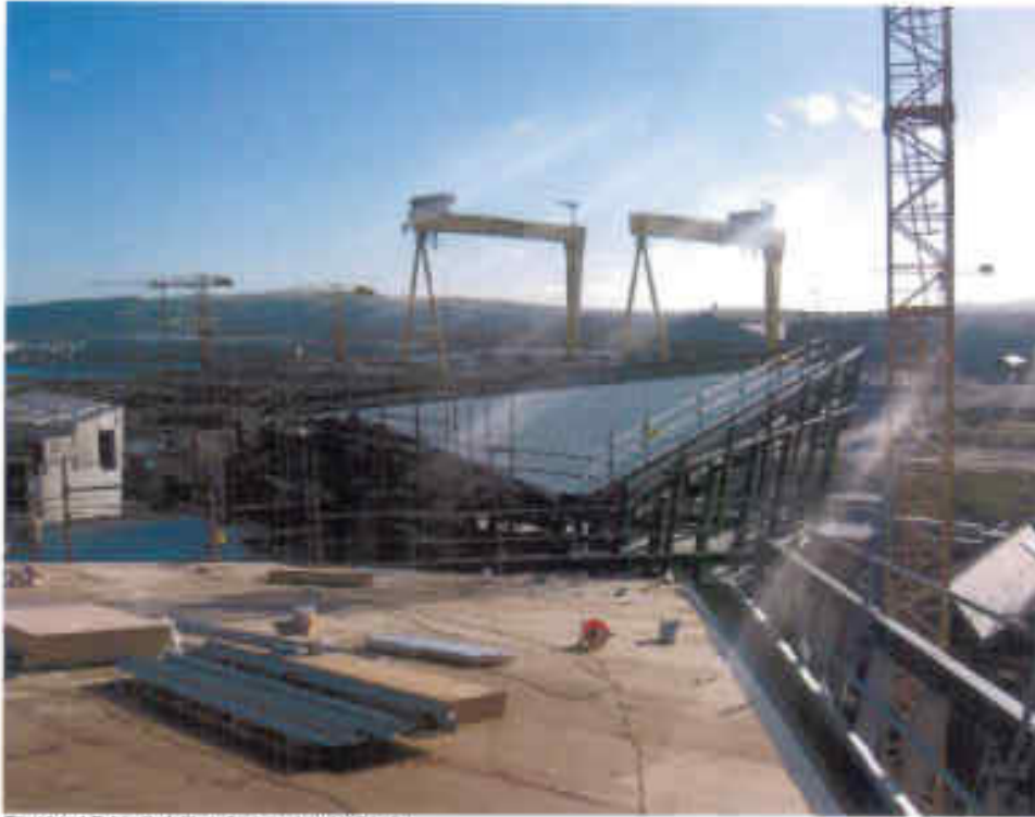
Photo 15 Hull 4 Roof (as at 30/9/10)
