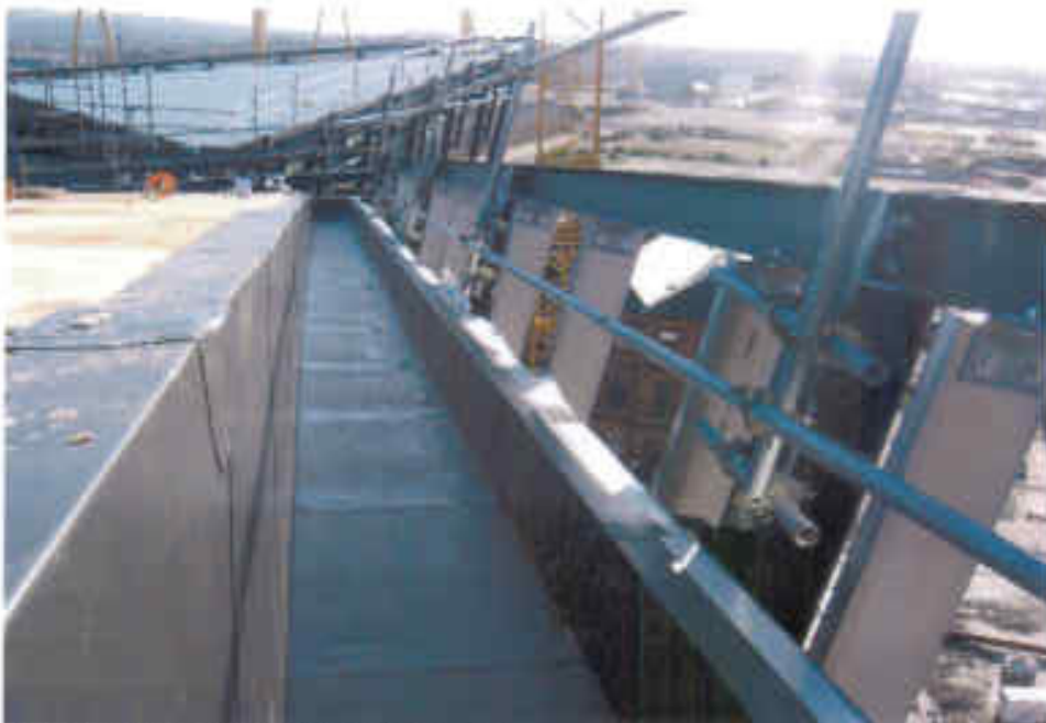
Photo 14 Hull 4 roof guttering (as at 30/9/10)
