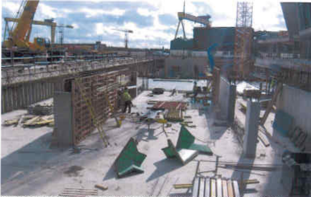
Photo 11: Outside Building Contract (NW Ramp in Construction from -1 to Ground) (as at 8/9/10)
