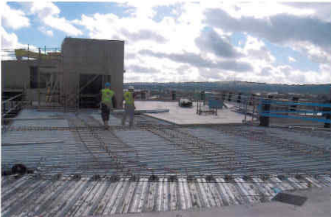
Photo 6: Hull 3 Metal Decking & Concrete Infill – Level 5 (as at 8/9/10)
