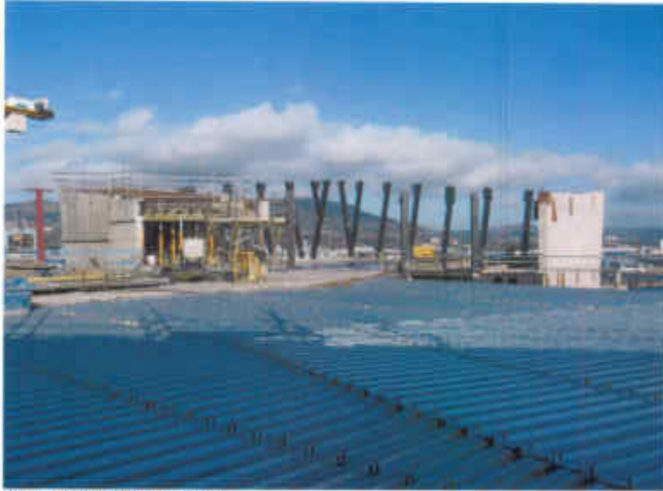
Photo 17 Roof view over Hull 1.
