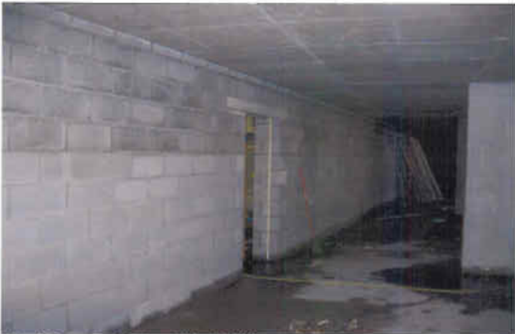
Photo 10: Basement – 2 Blockwork: (As at 8/9/10)
