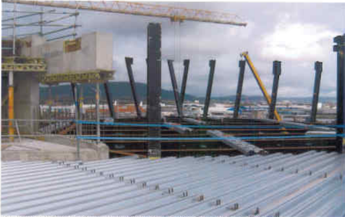
Photo 7: Hull 1 Structural Steel at roof (note: metal decking in foreground) (as at 8/9/10)
