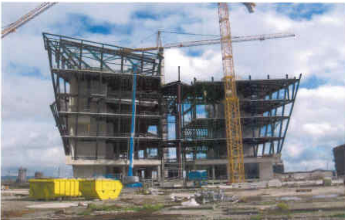
Photo 2: View of South Elevation (as at 8/9/10)
