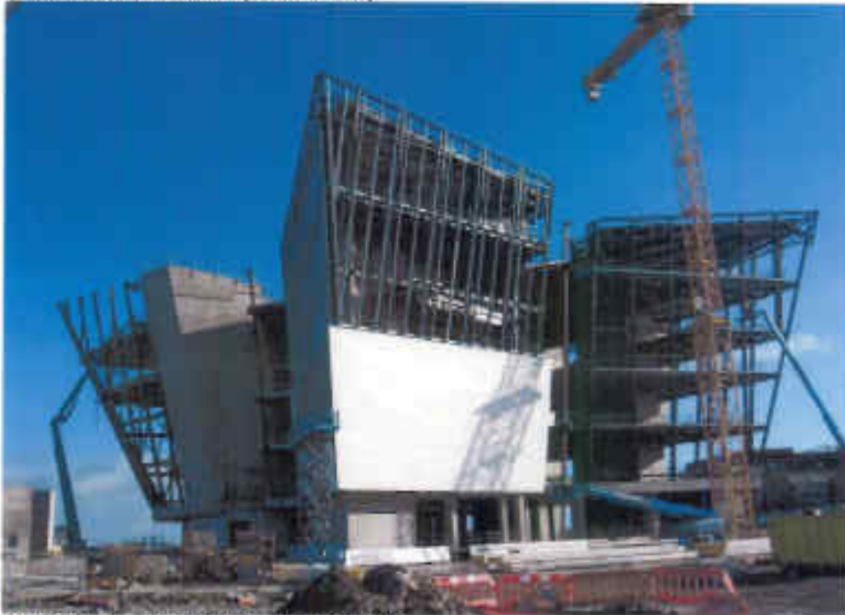
Photo 20 South West Corner (as at 30/9/10)
