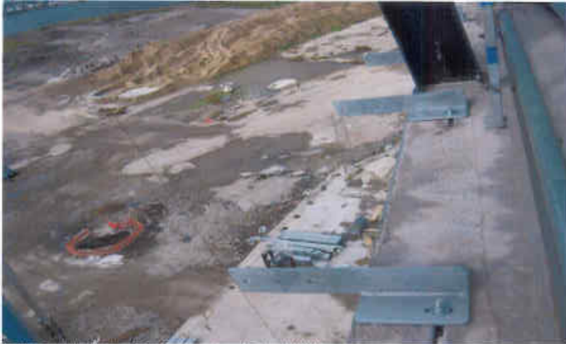
Photo 5: Hull 4 Cladding Rail Brackets – Level 5 (as at 8/9/10)
