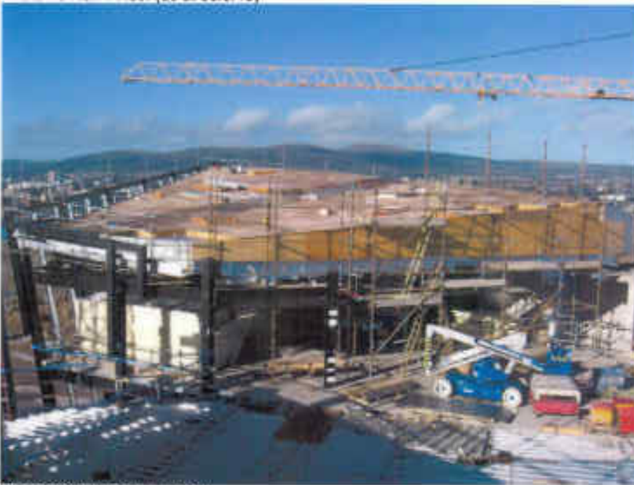
Photo 16 View of Hull 4 Roof
