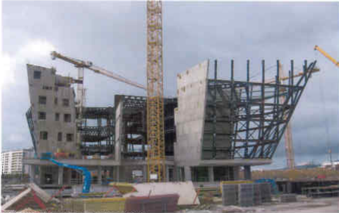
Photo 1: View of North Elevation (as at 8/9/10)
