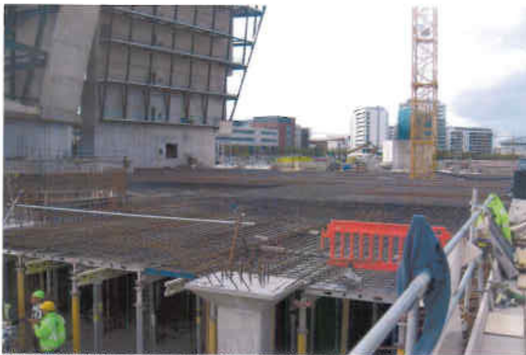
Photo 12: Outside Building Contract (Plaza Slab – West Elevation) (as at 8/9/10)
