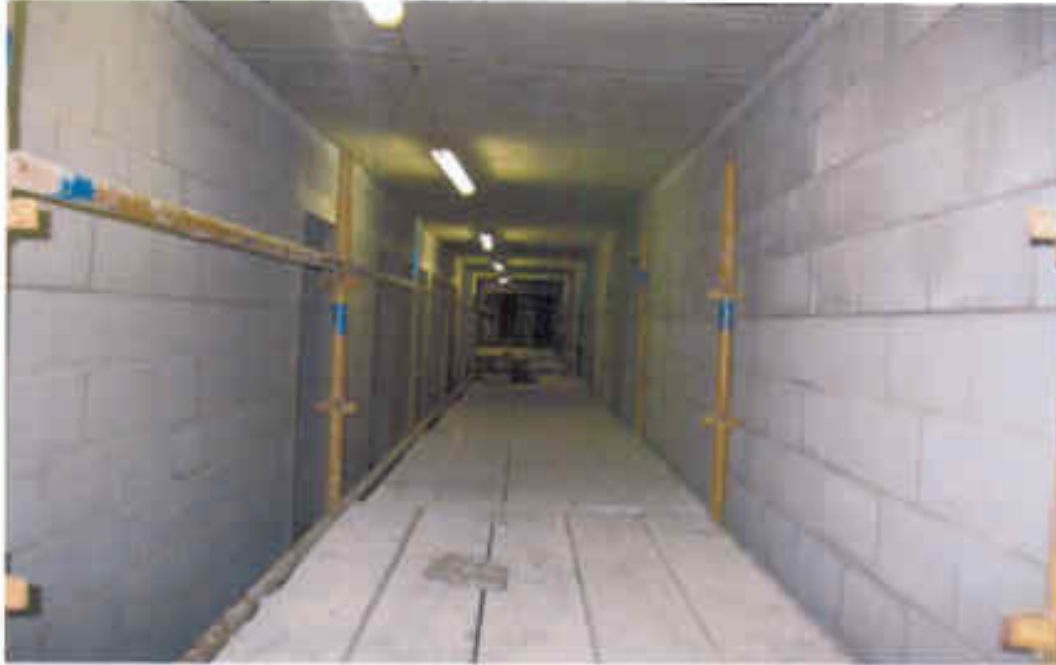
Photo 9: Basement -2 Blockwork – Circulation Corridor (as at 8/9/10)
